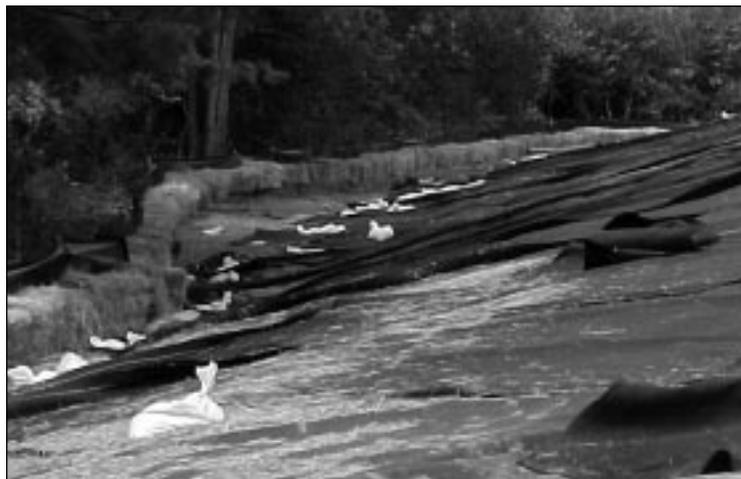
The closure of F Lot also involved placement of a flexible membrane liner (FML), as shown in this photo. The white sandbags hold the liner in place during construction. Hay bales visible along the perimeter are part of the stormwater detention system.
